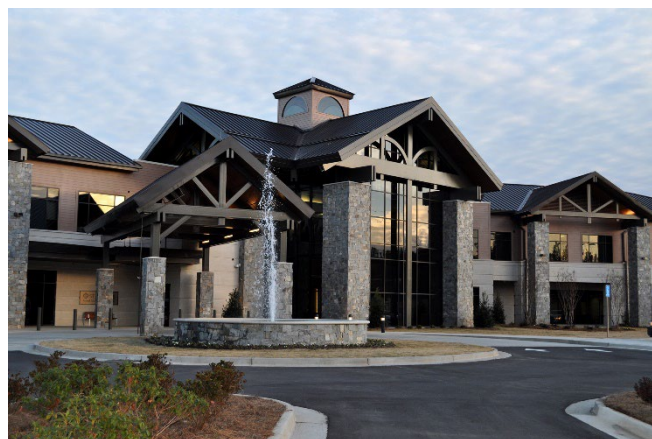
St. Mary's Good Samaritan Hospital, Greensboro
