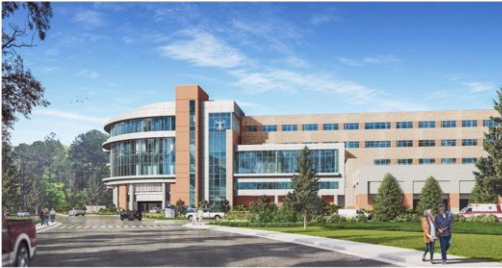
VIEW FROM THE CORNER OF N THORNTON AVENUE AND BURLEYSON ROAD
